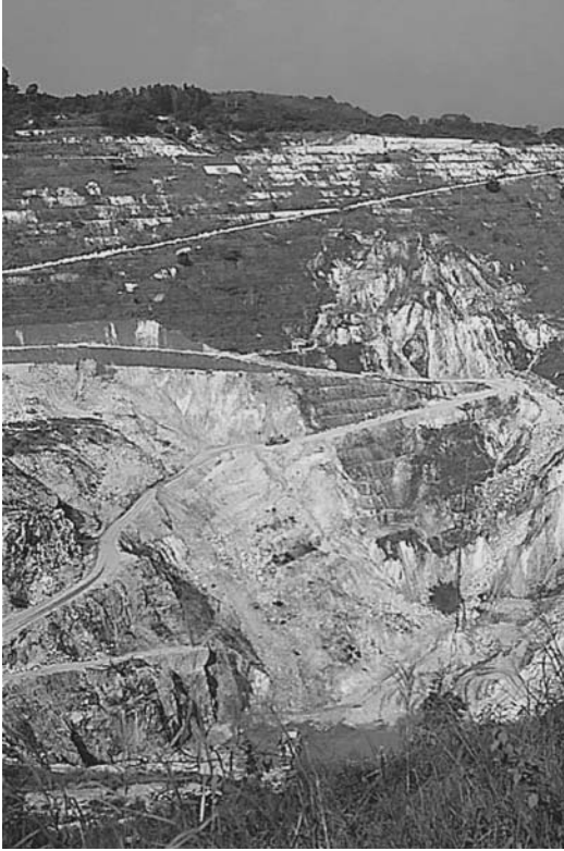
Figure 12.2 Sungai Besi tin mine, south of Kuala Lumpur, Malaysia. This is one of the world's largest holes in the ground (a large lorry mid-photo gives an idea of scale). Once worked out, the pit will flood. Spoil (sandy tin tailings) from mines in this region has caused considerable nuisance, choking streams and lying as an infertile layer over large areas.
