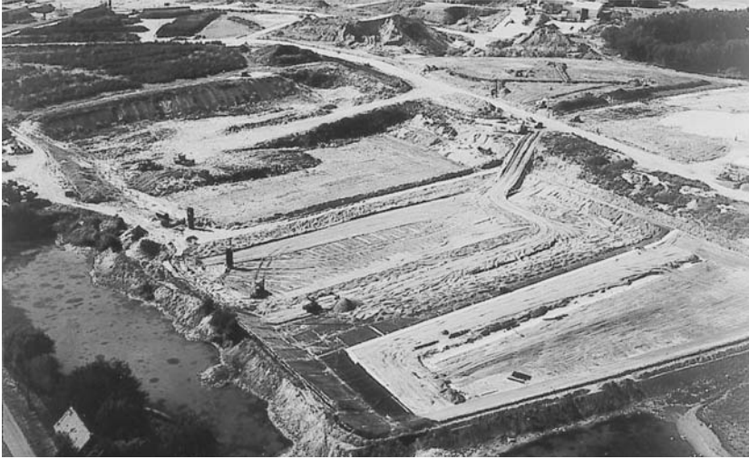
Figure 12.1 Landfill refuse disposal site in Belgium. This is a state-of-the-art facility with geosynthetic clay and high-density polyethylene lining to prevent leaching. Each pit can hold about 250,000 tonnes of waste. The gas emitted during decomposition is captured for electricity generation.
