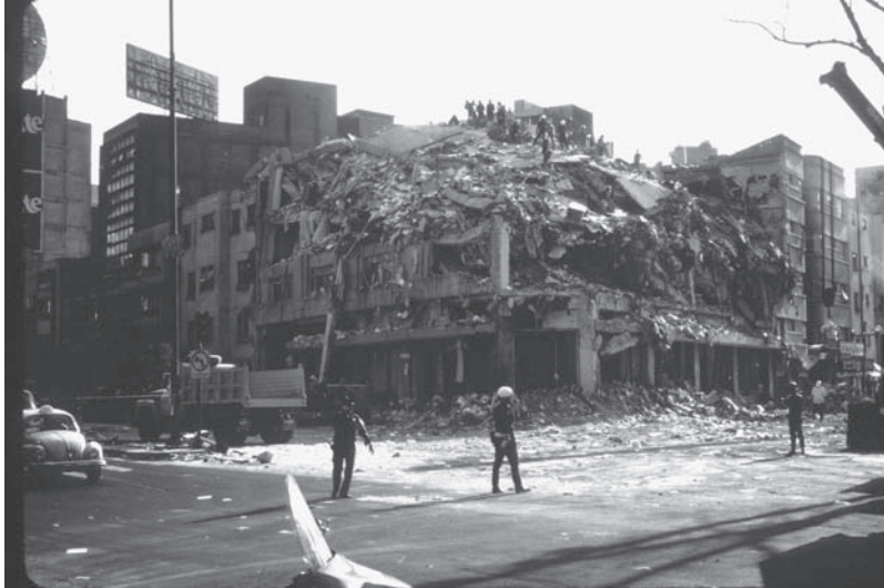
FIGURE 5–10 Mexico City Earthquake, September 19, 1985. The top floors of this eight-story building collapsed because of pounding against surrounding buildings. Available at: http://libraryphoto.cr.usgs.gov/htmlorg/lpb030/land/cel00012.jpg .
