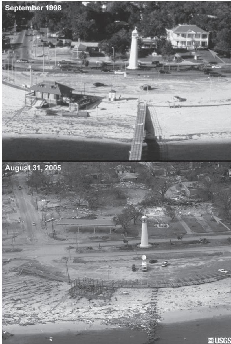
FIGURE 8-1 In the top image, taken in 1998, notice the pier, pier house, and the antebellum house in Biloxi, MS. The bottom image shows the same location on August 31, 2005, 2 days after Hurricane Katrina made landfall. This photo shows the complete destruction of these landmarks.
