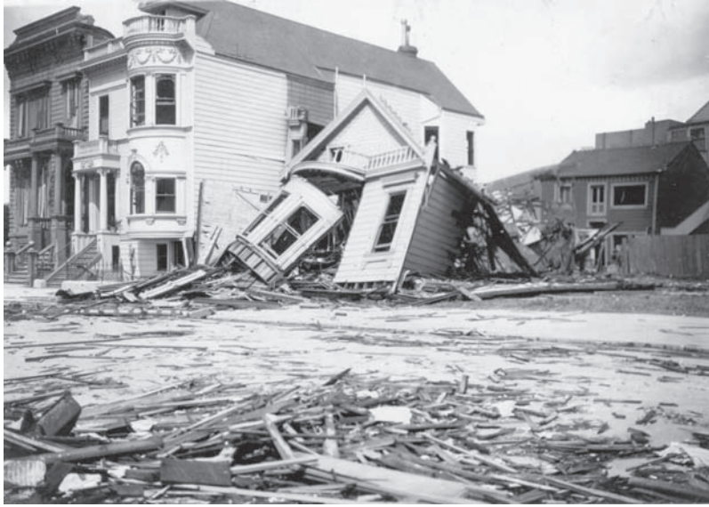
FIGURE 5–2 San Francisco, California, Earthquake, April 18, 1906. Ruined house on Shotwell Street. Photo courtesy of U.S. Geological Survey. http://libraryphoto.cr.usgs.gov/html/lib/batch01/batch01j/batch01z/batch01/ggk02894.jpg .
