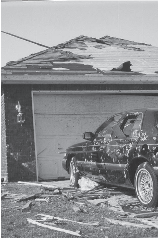
FIGURE 11-3 Tornado damage from a 1999 Oklahoma City tornado. Note the board driven through the car door.
