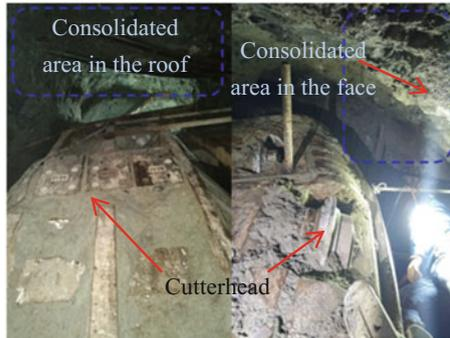
**Fig. 8.** The surrounding rock after grouting near the cutterhead
