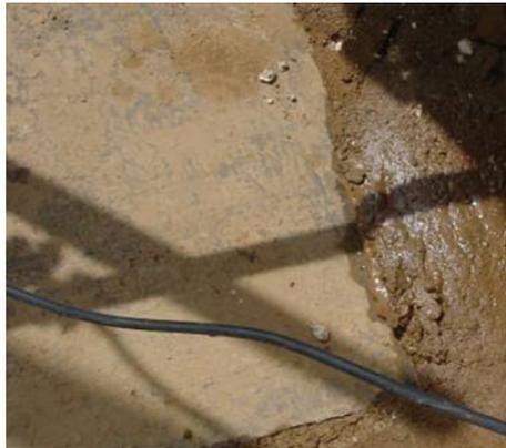
**Fig. 6.** Mud-pumping of subsoil
