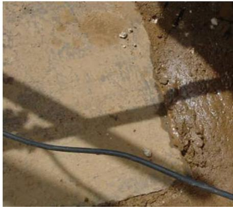
**Fig. 6.** Mud-pumping of subsoil
