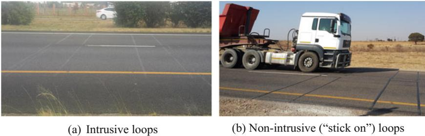
**Fig. 1.** Typical intrusive and non-intrusive loop systems
