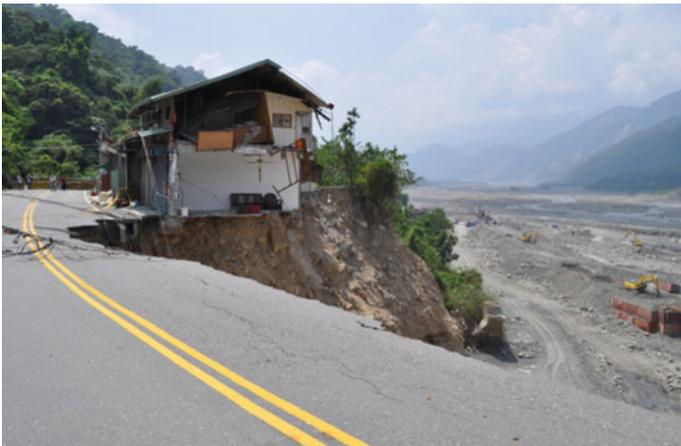
**Fig. 2.** Downslope of Shin-Shan Village collapsed and near fallen houses beside the river
